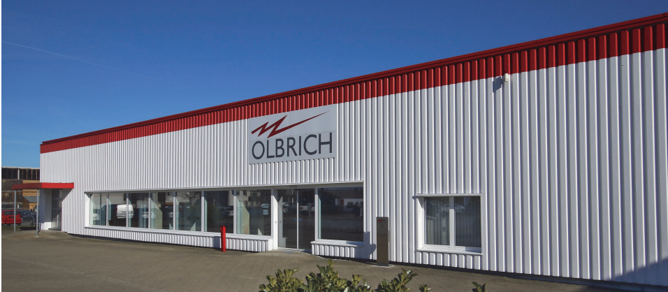
Innovationshalle in Goslar
